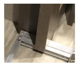
You will need to cut a notch into the bottom of the sliding bathroom door to allow the rack to slide in under it. This holds this corner of the rack down.
